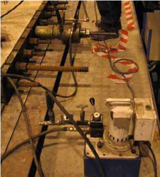
Figure 4.14 Equipment for post-stressing the Dywidag bars.
