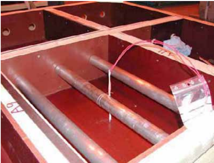
Figure 3.3 Mould with pipes for post-stress bars and installed thermocouples.
