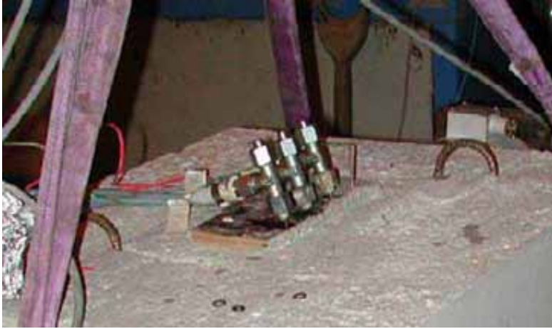
Figure 4.5 The pressure gauges connected to the small pipes with angle tees.
