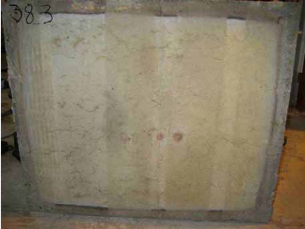
Figure A.336 Specimen 38-3 after test.
