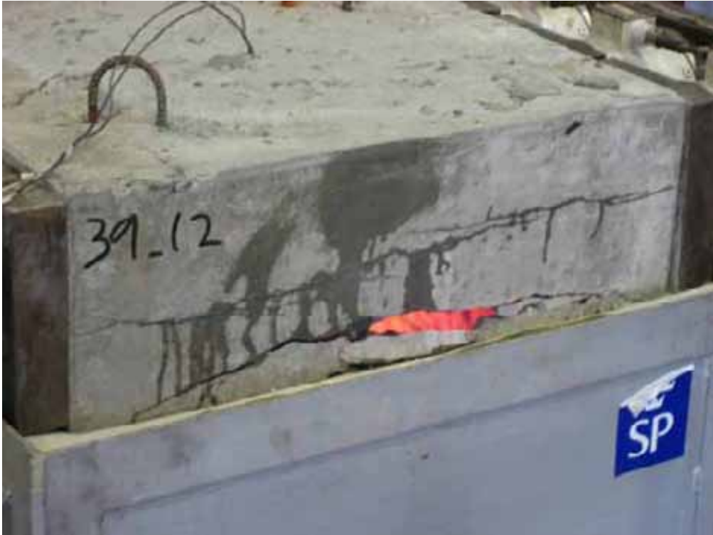
Figure A.344 Specimen 39-12 during the test. It has spalled through the side.
