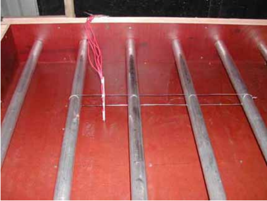
Figure 3.9 Aluminium tubes mounted in the mould as well as a wooden stick with thermocouples.
