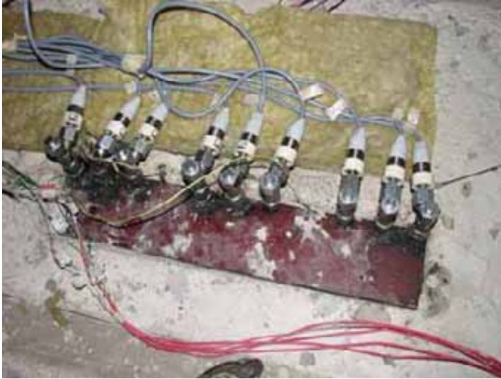
Figure 4.17 Pipes connected to pressure gauges.
