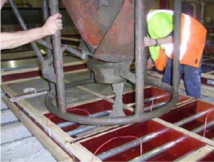
Figure 3.4 Casting of small slabs.
